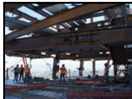
Structural Steel Erection
