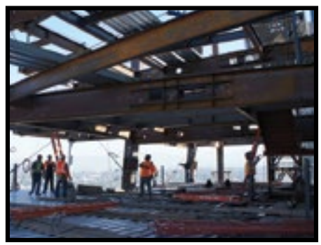
Structural Steel Erection
